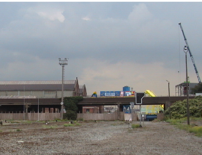
Dam viaduct + WDT
